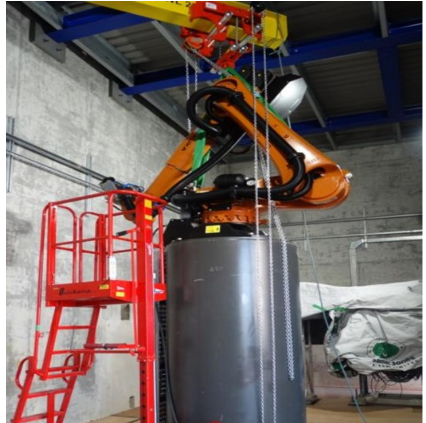
Installation of Kuka robot onto its pedestal
