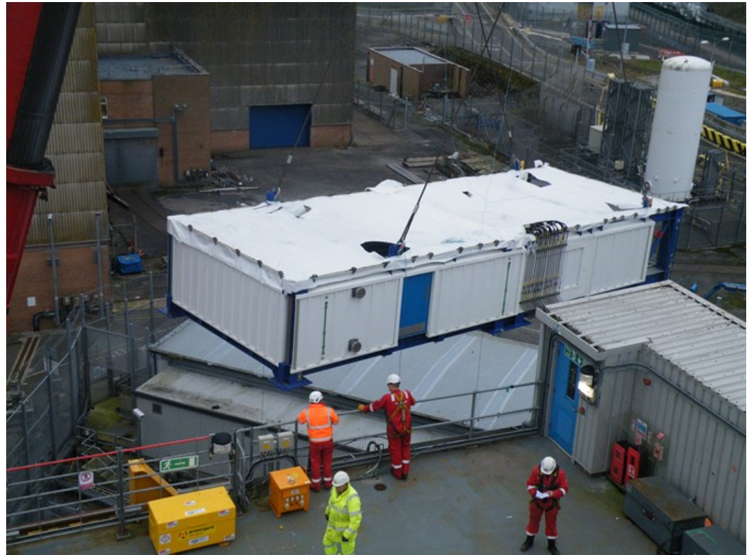
Waste Container Transfer Area Module Installation
