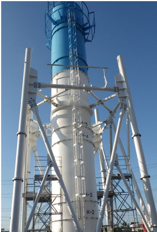
Stack mock-up built on the premises of ABLE with the same size as the upper portion of the stack
