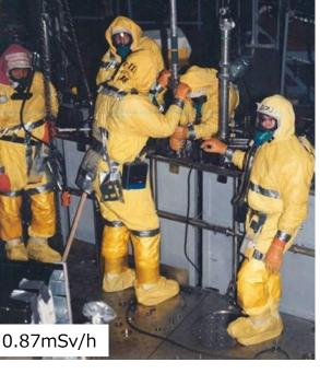
A state of removing fuel debris
