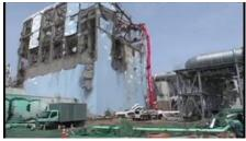
Water discharge to spent fuel by concrete pump car
